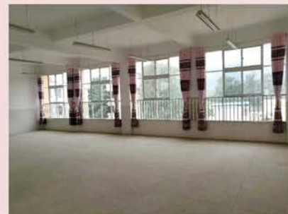
Classroom before construction
